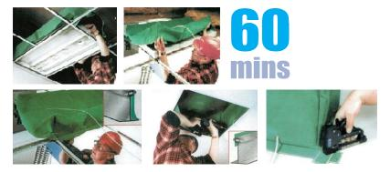
Fireus Canopies and Downlight Coves are designed specifically to stop the passage of smoke and fire through a fire-rated ceiling, where recessed luminaires or downlights are fitted.
